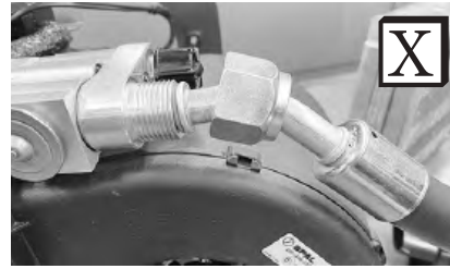
Improperly Seated O-ring Land
