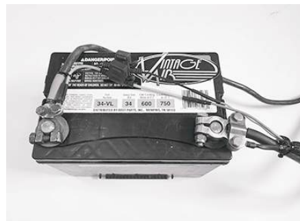
Completed Installation Shown
